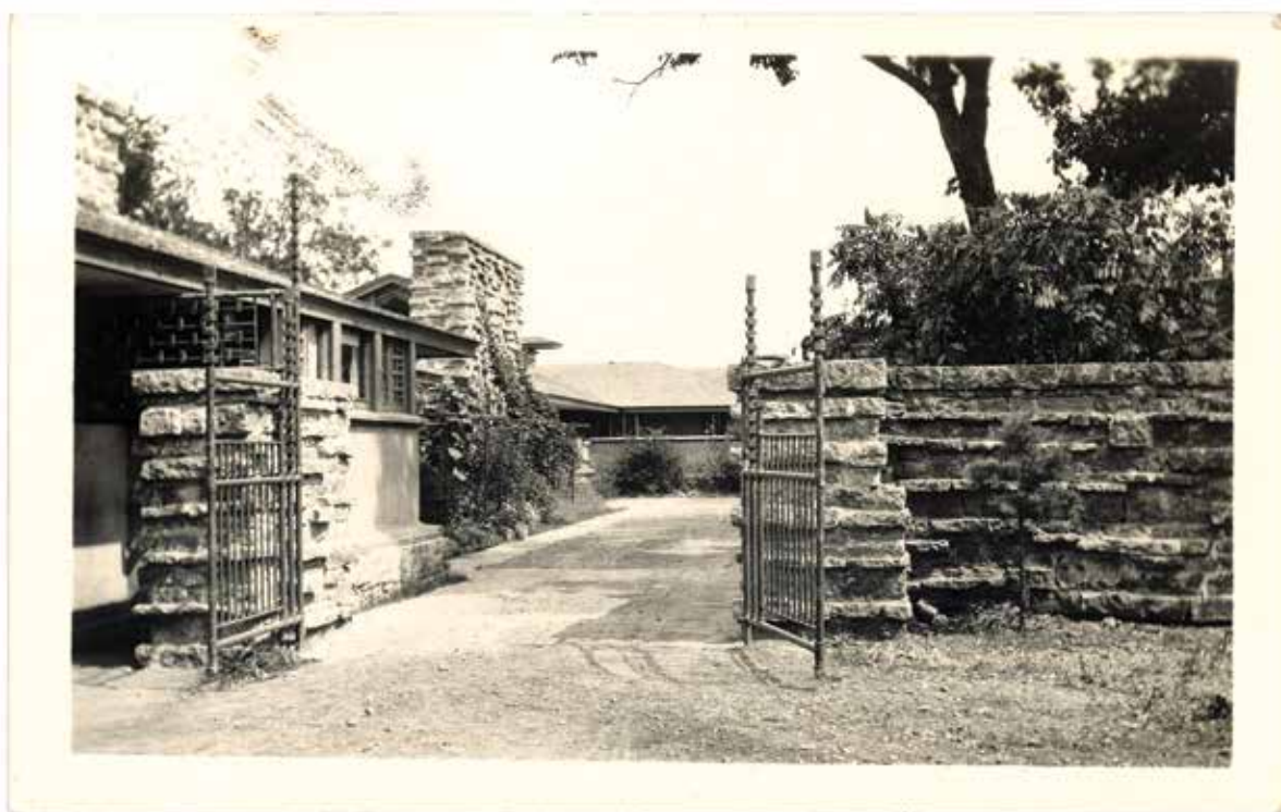
This is a 1912 view into the Taliesin courtyard in Spring Green. The gates were formed with pipe railing sections and located within an opening in the limestone wall.
