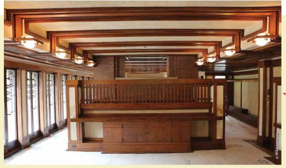
raised ceiling which folds down upon the horizontal band resting above the series of glass door and window openings which provide a spatial release to the outside. With Wright, it is not either enclosure or openness, but both/and. Even fine details such as the stained glass window patterns delicately reinforce spatial enclosure while also allowing views and light to pass through. His synthesis is to hold onto both ideals and find a way to realize them together.
