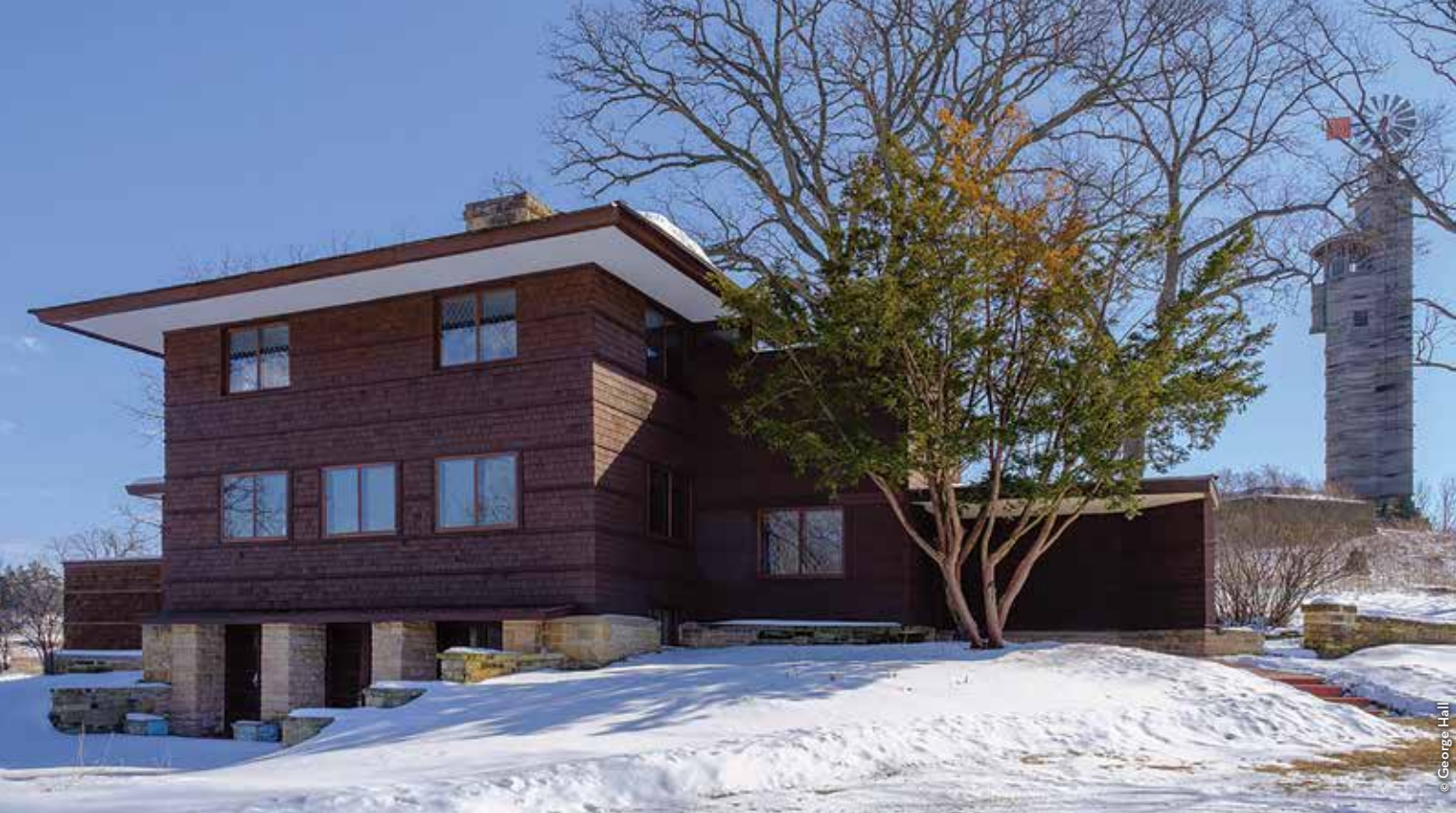
Recently restored, Tan-y-Deri on the Taliesin estate dates from 1907. Frank Lloyd Wright designed it for his sister Jane and her husband William Porter, associated with the Hillside School.
